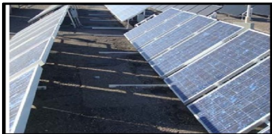
Fig. 5. Inter-row or self-shading of PV module in field conditions (Picture source [38]).
